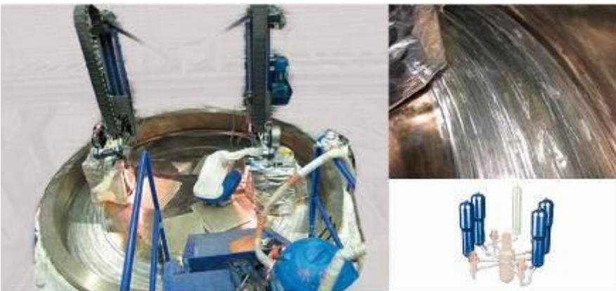
*Fig. 14: Deposit of a protective coating on a steam generator tube sheet (cladding operation)*
